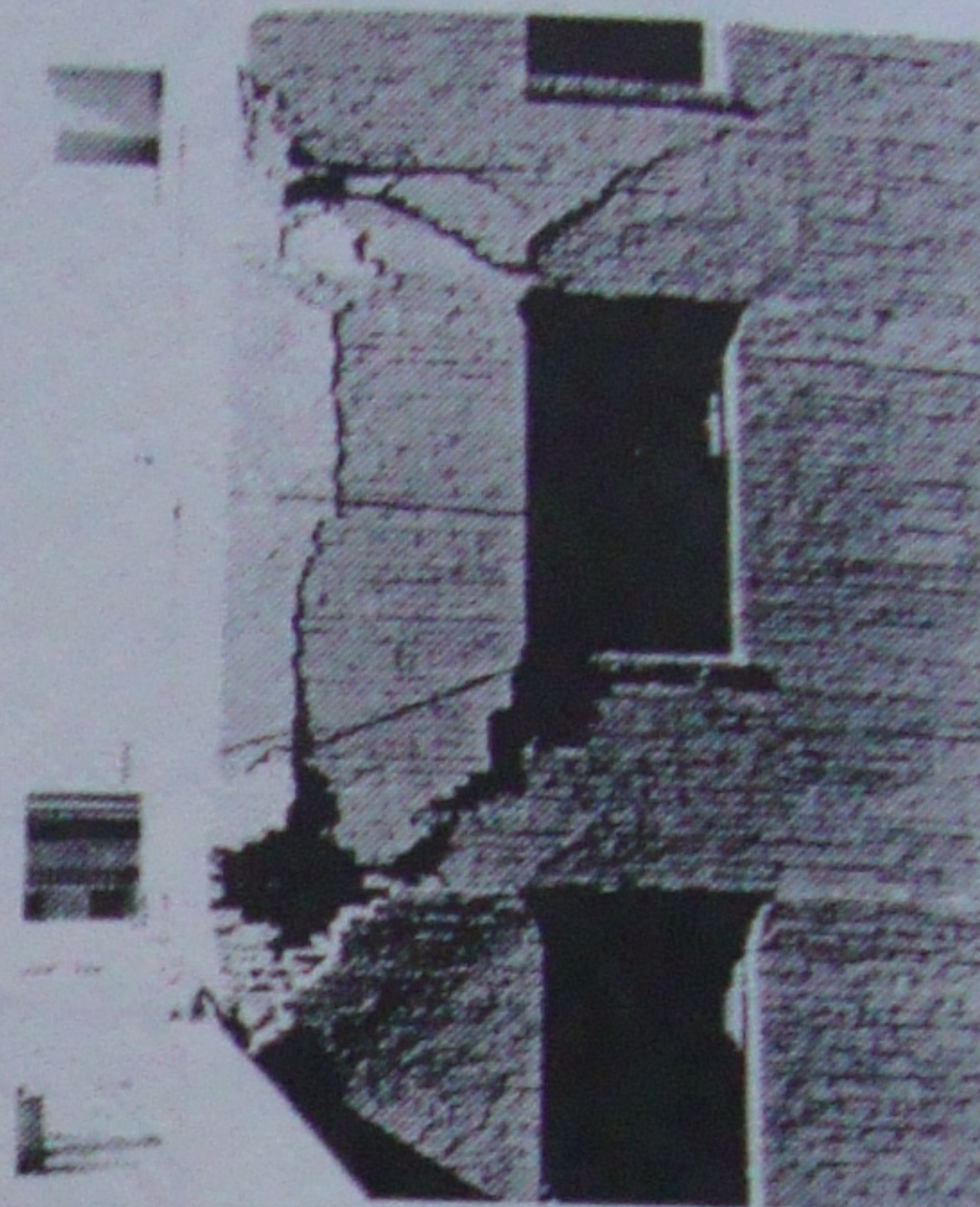
Fig. 7 Example pounding damage (13th Street, Oakland City Center)
