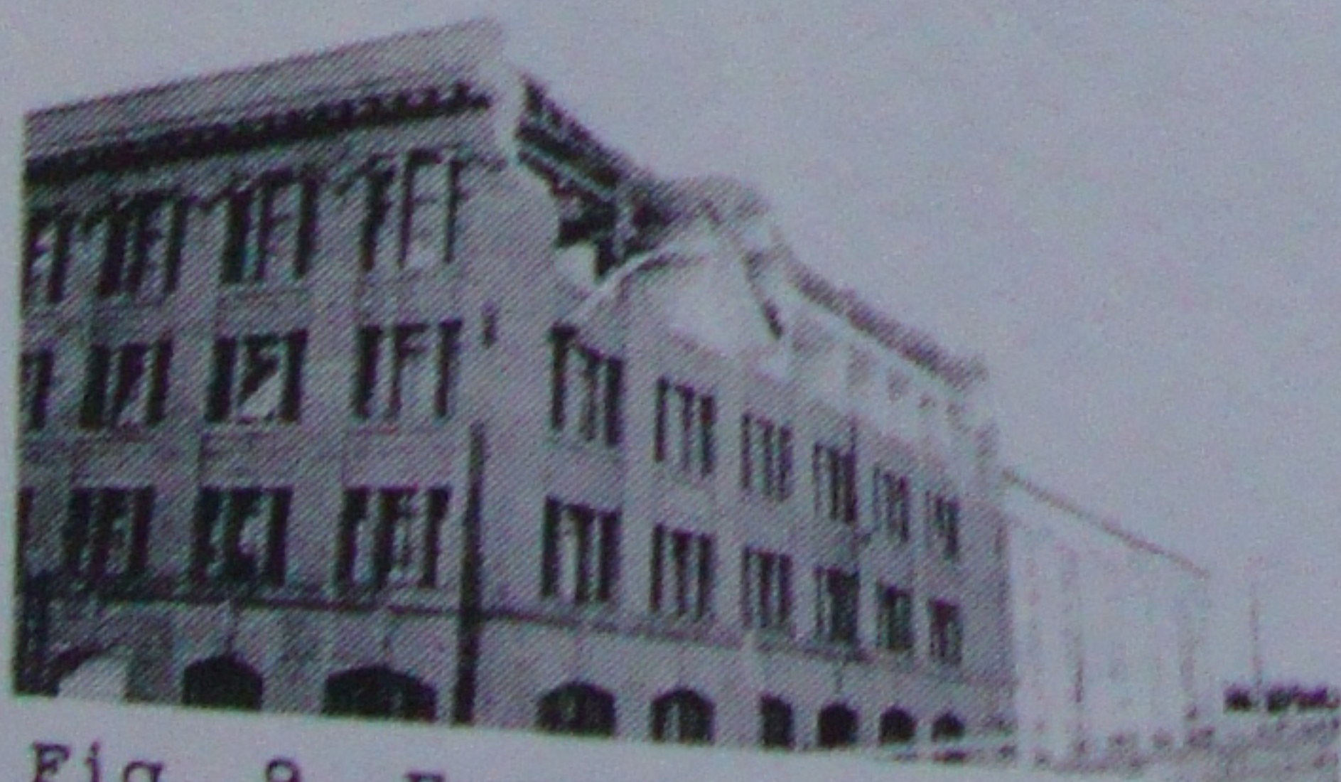
Fig. 8 Example pounding damage (11th Street, Oakland City Center)
