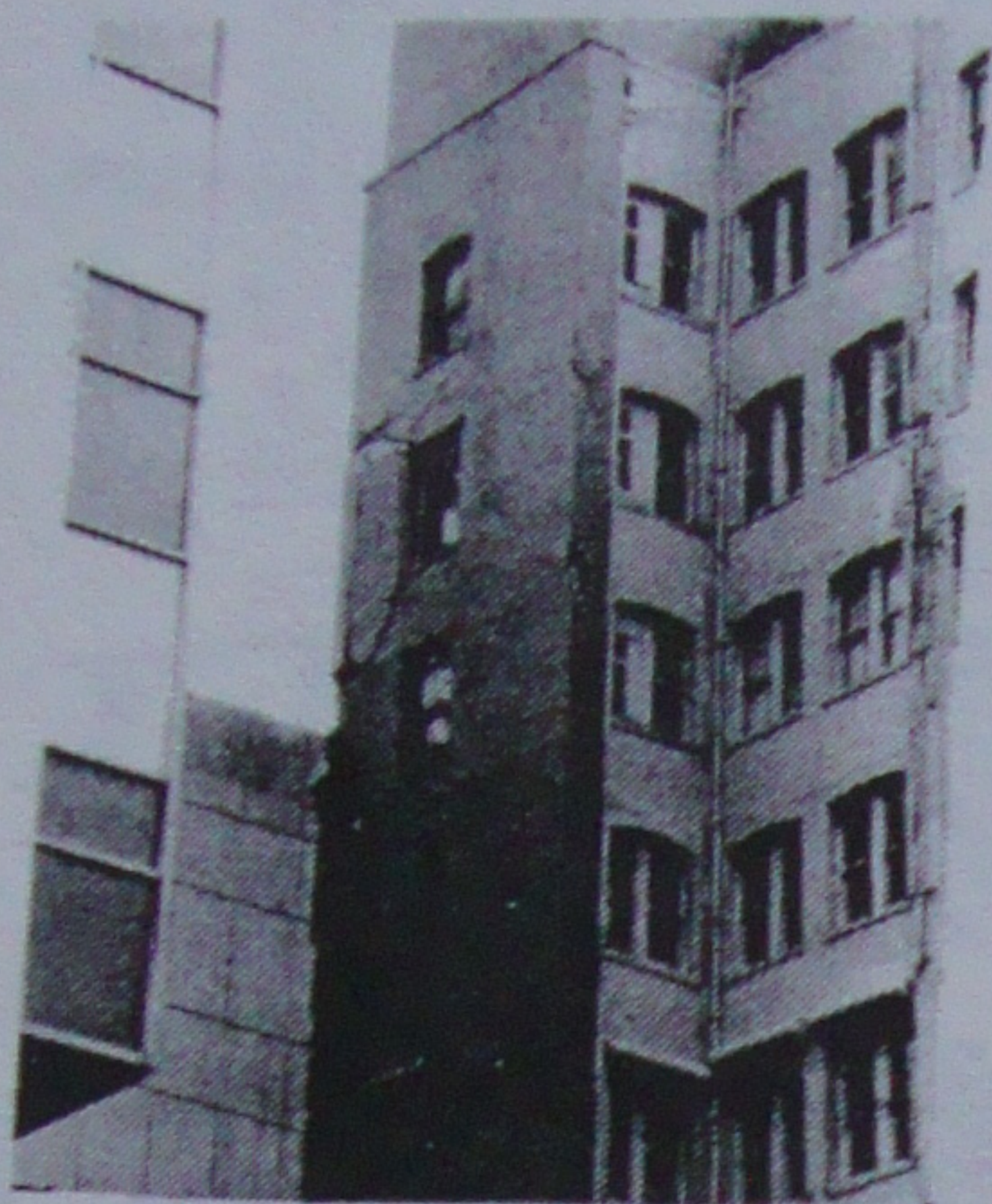
Fig. 7 Example pounding damage (13th Street, Oakland City Center)
