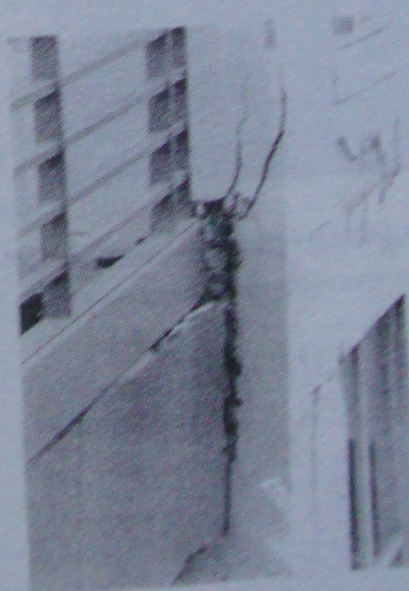
Fig. 5 Example pounding damage (Broadway Street, Oakland)
