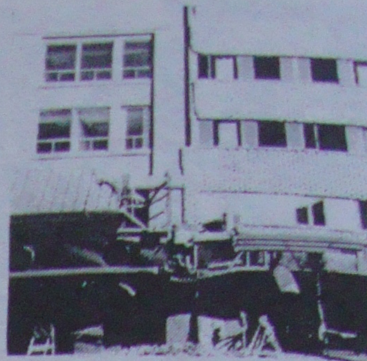
Fig. 6 Example pounding damage (Franklin Street, Oakland)
